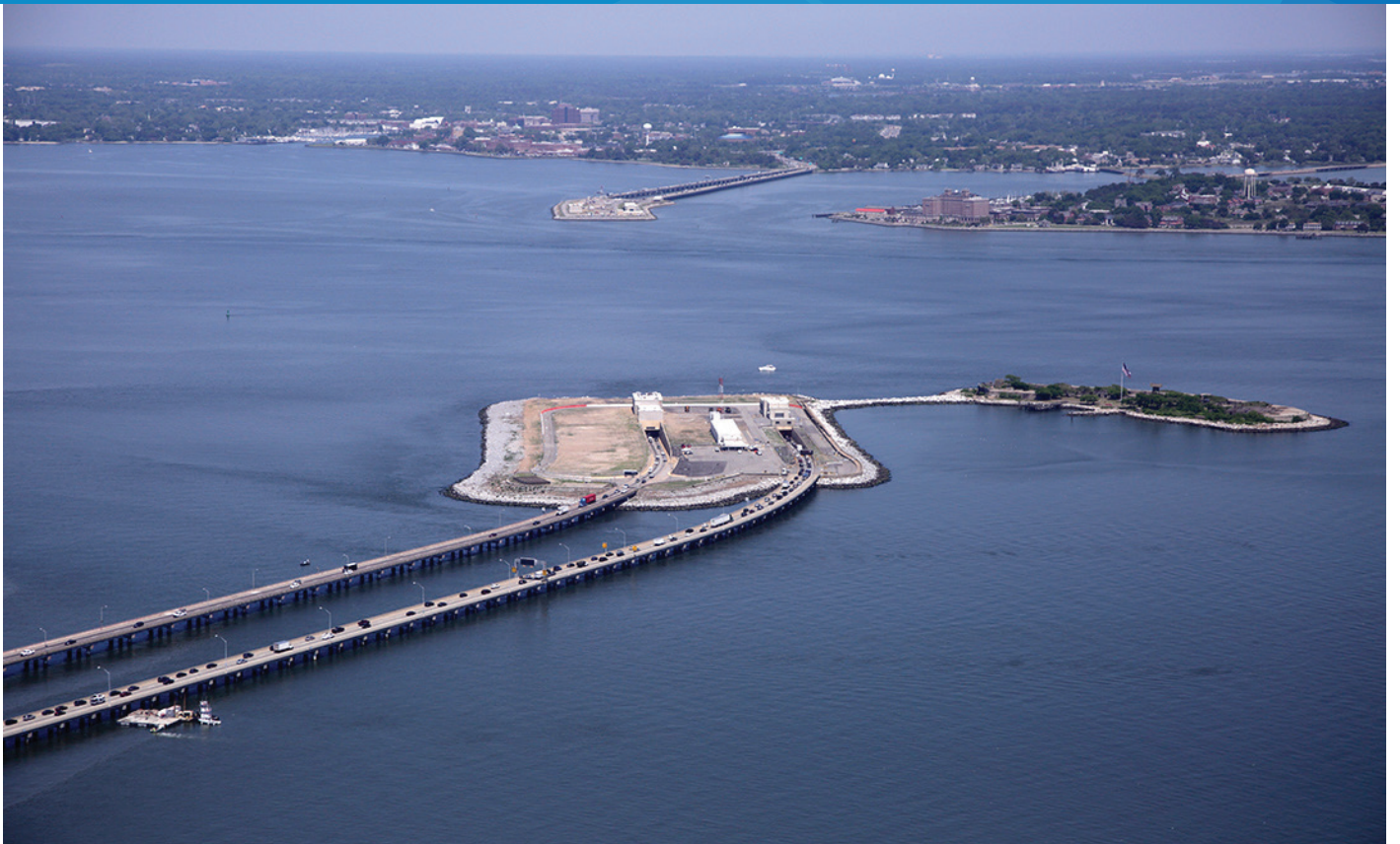
▶ This photograph shows the structures leading to the tunnels and open shipping channel.
