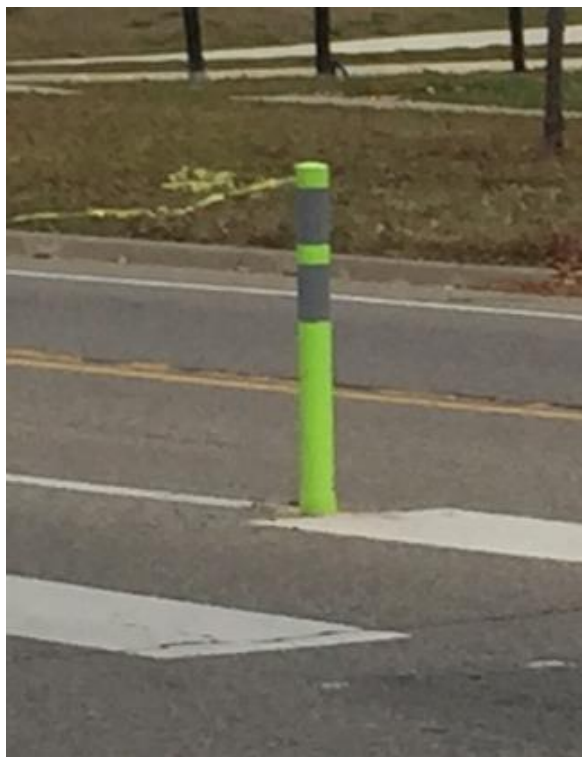
Figures 2a-c. Figure 2a (above left) shows an R1-6 sign installed on a removable curb base. Figure 2b (middle) shows a flexible delineator installation. Figure 2c (above right) shows an R1-6 sign mounted on a flush mounted base.
