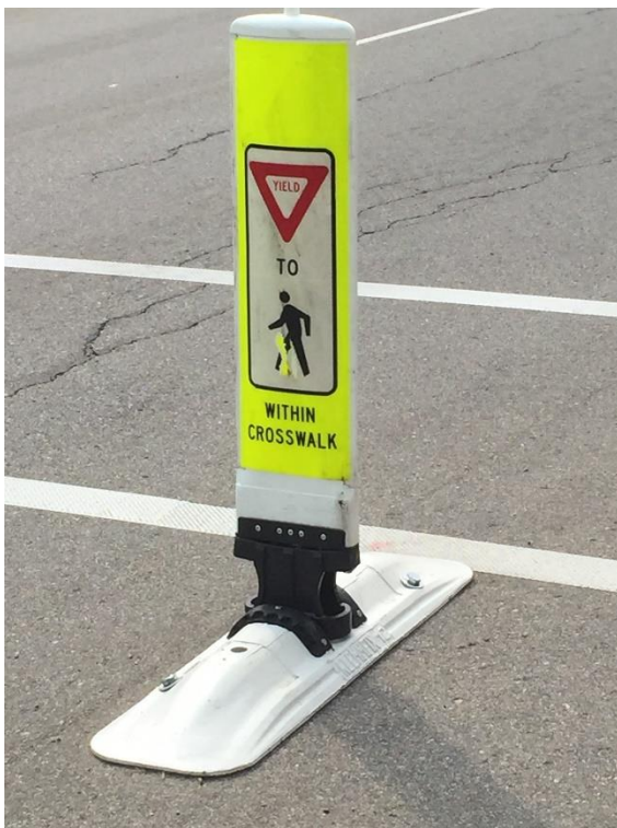
Figures 2a-c. Figure 2a (above left) shows an R1-6 sign installed on a removable curb base. Figure 2b (middle) shows a flexible delineator installation. Figure 2c (above right) shows an R1-6 sign mounted on a flush mounted base.
