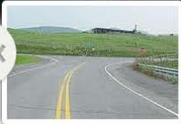
Roadway Condition Data
