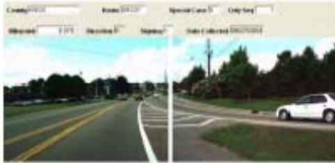
Photo 1. TRIMS Image looking northbound where the Ramp from SR-33/Broadway enters at L.M. 0.11.
