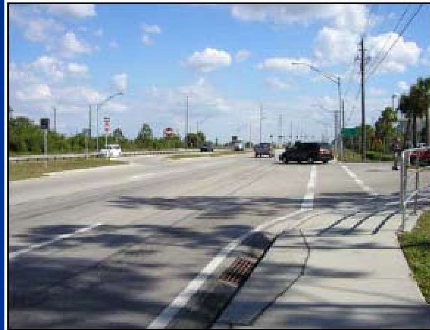
access and left-in median break for the "Shoppes of Pebblebrooke" shopping mall
