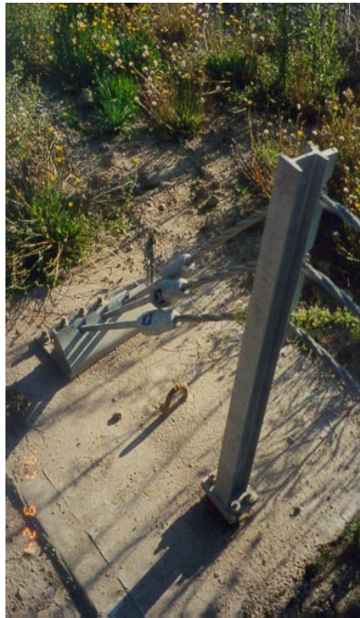
Figure 2.5: Anchor post slip base and concrete footing
