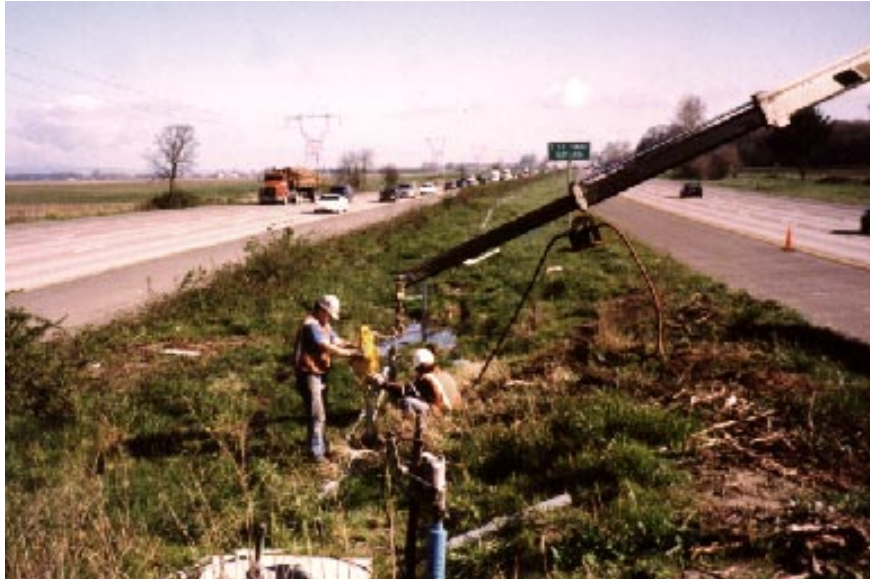
Figure 4.2: Installing new steel posts
