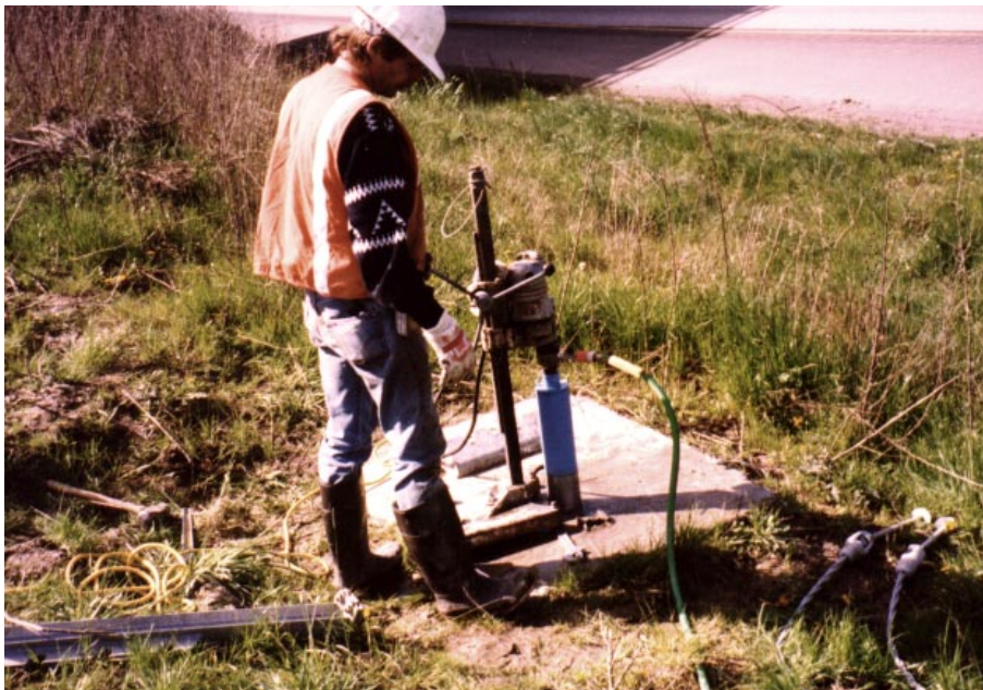
Figure 4.3: Coring a new hole for a replacement anchor post
