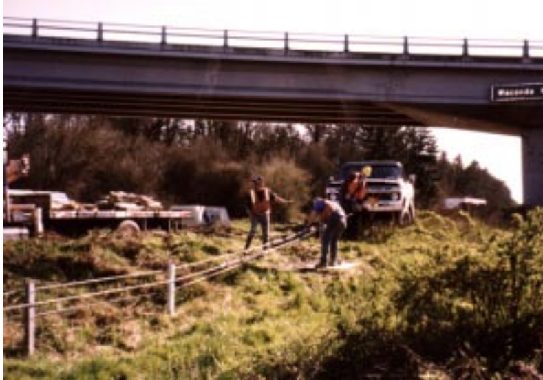
Figure 4.4: Stretching the reattached cables
