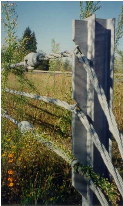
Figure 2.4: Anchor post bracket with 3mm tabs
