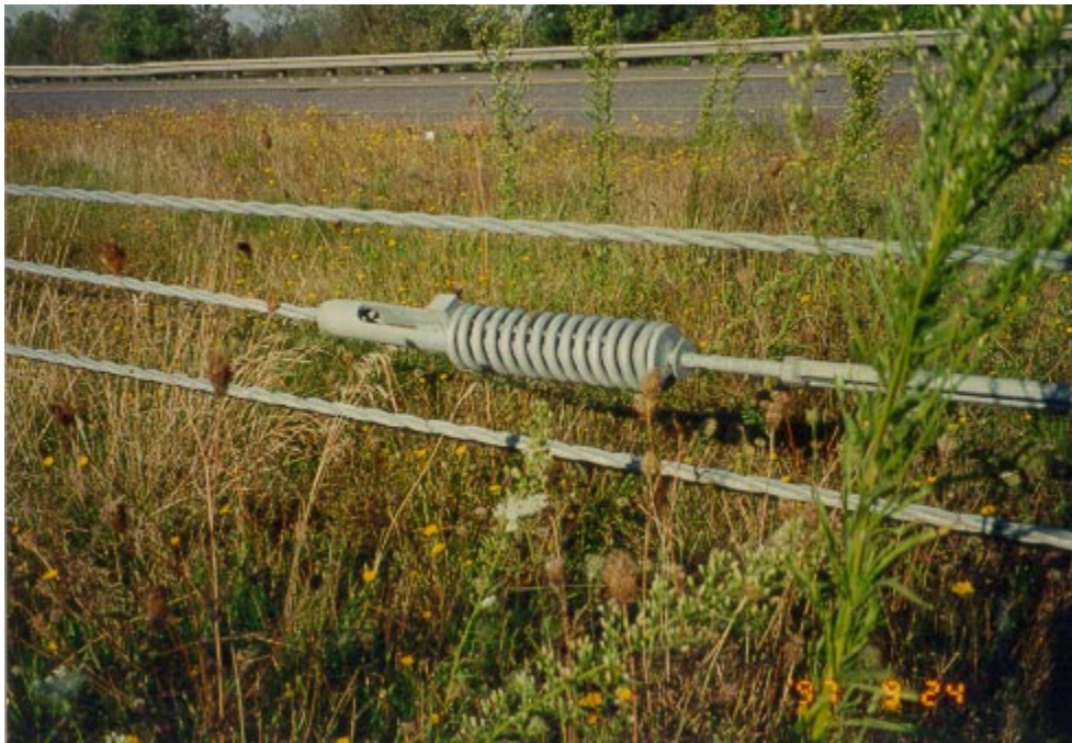
Figure 1.1: Three-cable median barrier system with spring turnbuckle
