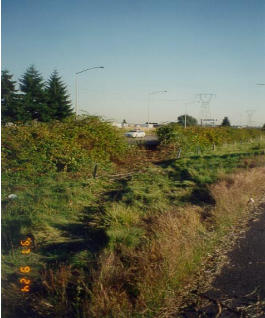
Figure 3.2: Semi-truck crossover through cable median barrier
