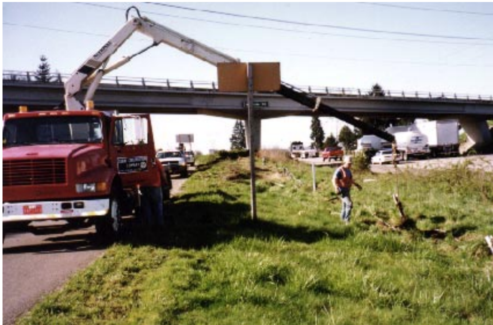
Figure 4.1: Removing damaged steel posts
