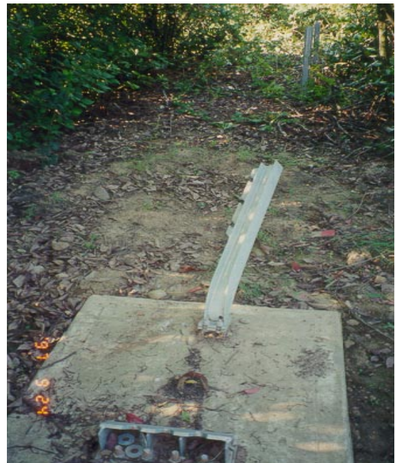
Figure 3.5: Energy dissipation-cable release from breakaway anchor angle and anchor post bracket (north end)
