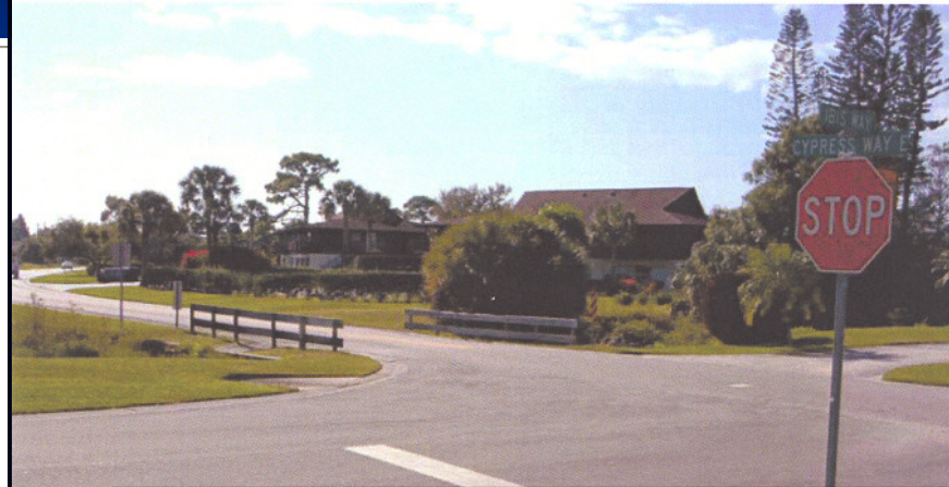
Figure 1. Culvert at Intersection of Cypress Way East and Ibis Way
