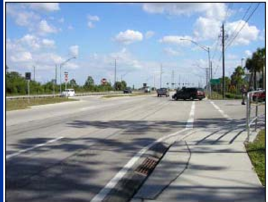
access and left-in median break for the "Shoppes of Pebblebrooke" shopping mall
