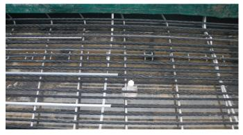
Prestressed concrete box beam casting bed with the CFCC strand, strand debonding plastic sleeves, and the bottom stainless steel U-rebars used for shear reinforcement installed in place near the beam end.
