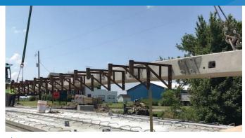
An exterior box beam being launched to set onto the beam seat.
