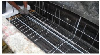
Prestressed concrete box beam casting bed with the CFCC strand and the bottom stainless steel U-rebars used for shear reinforcement installed in place. Note the bond breaking plastic sleeve being installed.
