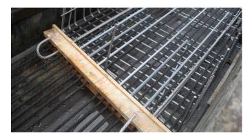
Looking at beam end of the prestressed concrete box beam casting bed with the CFCC strand and the bottom stainless steel U-rebars used for shear/confinement reinforcement installed in place.
