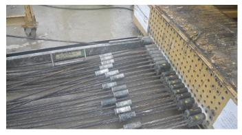
Prestressed concrete box beam casting bed with the bulkhead and prestressting chucks set in place color coded for the stressing operation sequences. Note the stressting jack will fit between two chucks to normally function.
