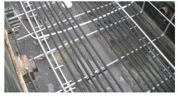
Prestressed concrete box beam casting bed with the CFCC strand and the bottom stainless steel U-rebars used for shear reinforcement installed in place. Note the rectangular block out at the lower left side of the photo of the exterior beam used to run the tie rods through beams during the bam installation operation.
