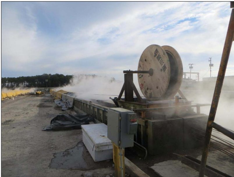
CFRP piles being steam-cured after stressing of the strands and concrete placement. A spool of CFRP strand can be seen above the stressing bed.
