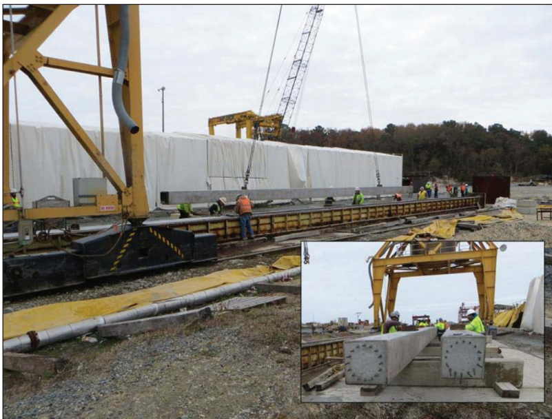
CFRP piles being removed from the forms and inspected.
