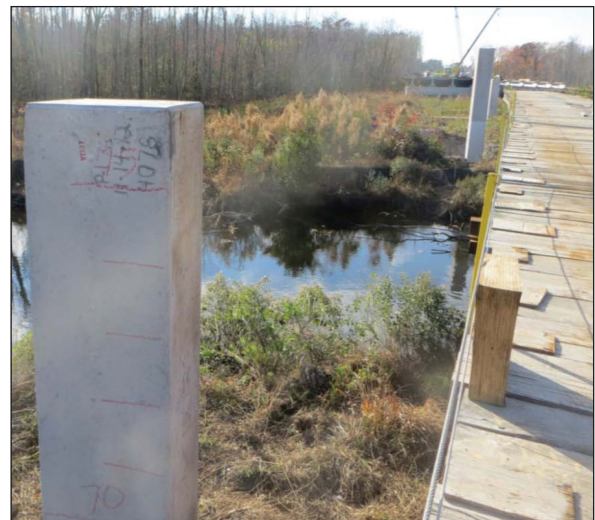
Corrosion-free CFRP piles adjacent to West Neck Creek after restrike and redrive, with a final elevation of 61'.
