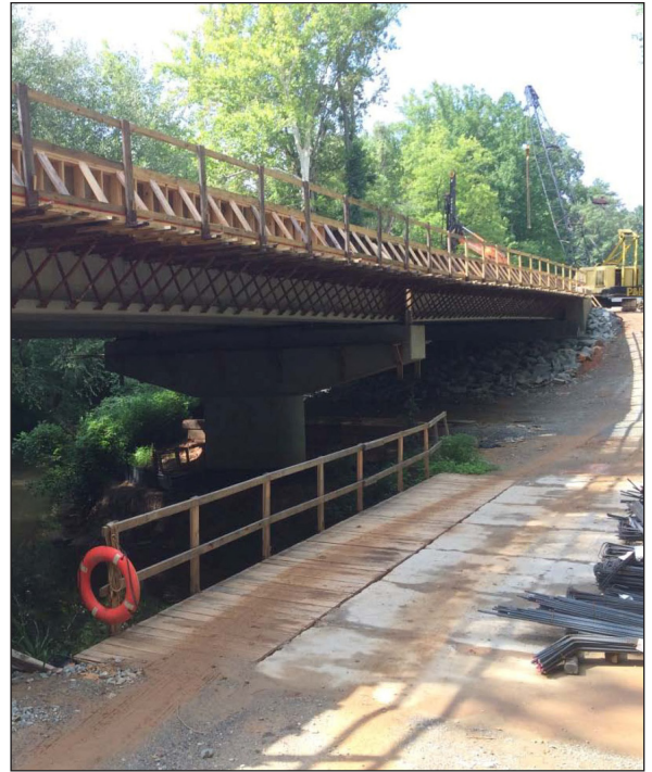
Deck work at jobsite with all eight CFRP beams in place.
