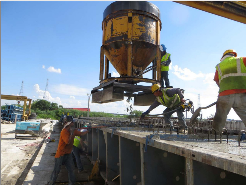
Placement of concrete during fabrication of CFRP beam.
