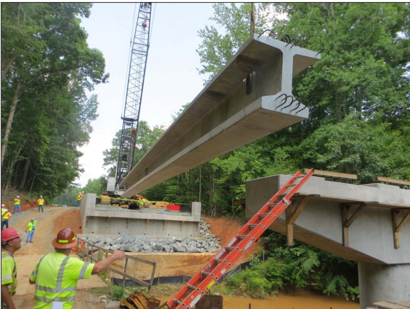
Placement of corrosion-free CFRP beam at jobsite.
