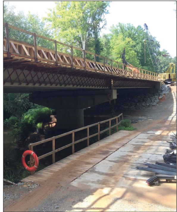
Deck work at jobsite with all eight CFRP beams in place.
