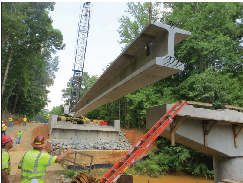
Placement of corrosion-free CFRP beam at jobsite.
