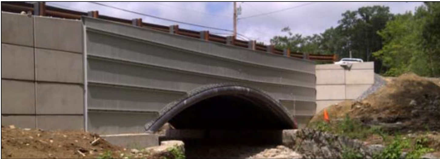
Scott Reservoir Outlet Fitchburg, MA
