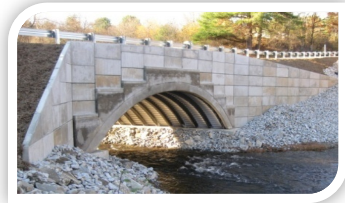
Royal River Bridge Auburn, ME
