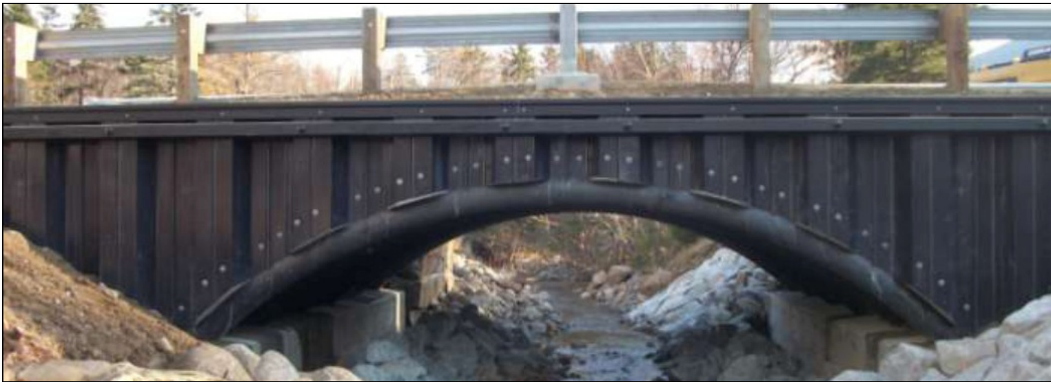
Pinkham Notch, NH 24' Span Composite Panel Headwall 6 Arches (12" Diameter)
