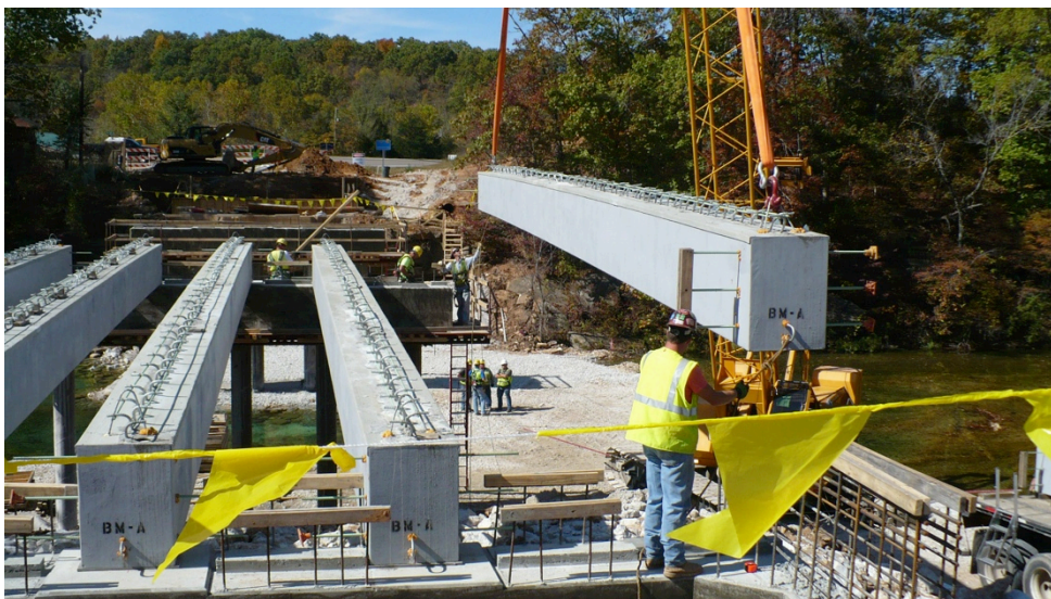
FIGURE 4.52 Setting pre-filled HCB's in on substructure
