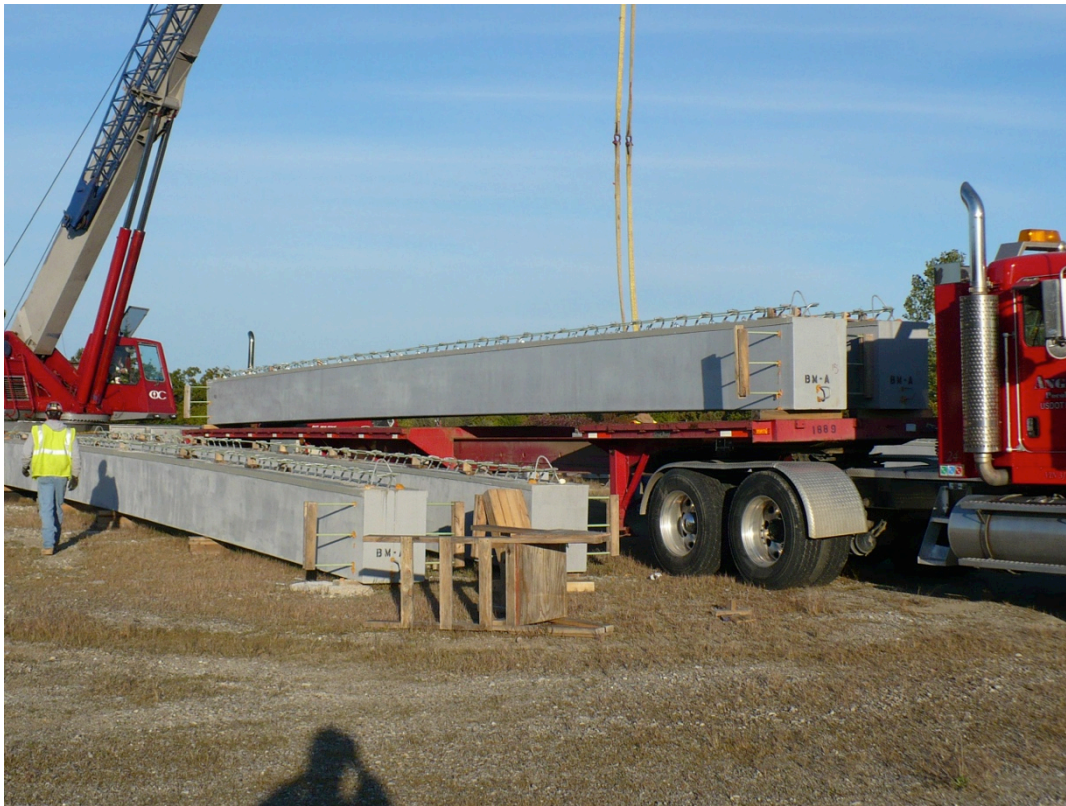
FIGURE 4.1 HCBs in staging yard prior to shipping to bridge site
