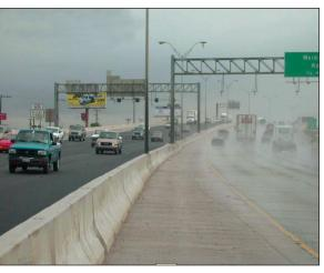
The use of permeable friction course (installed on the roadside to the left) reduces splash and spray.
