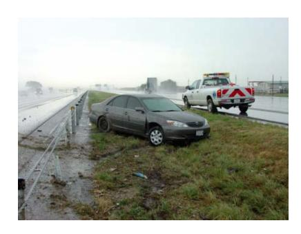
**End Cable Barrier Behind W-Beam**
