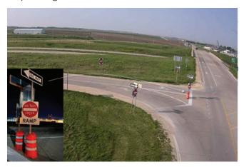
Enhanced signage (change left turn arrow to straight arrow in advance of exit ramp) – 76% reduction in wrong way driving events
