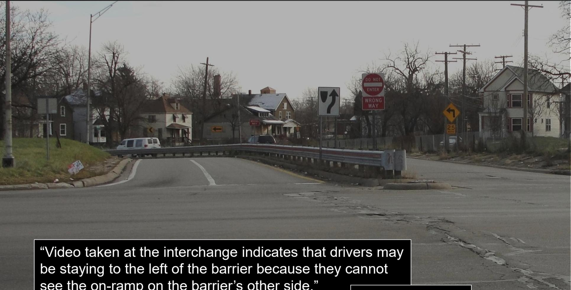
“Video taken at the interchange indicates that drivers may be staying to the left of the barrier because they cannot see the on-ramp on the barrier’s other side.”
