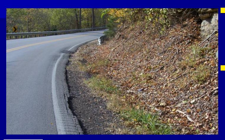
Shoulder drop offs in curve along entire route Excavate existing shoulders, replace with 4' paved shoulders w/ rumble strips
