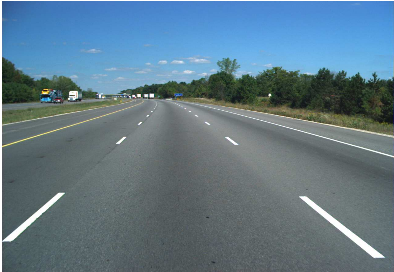
Depressed Median with 2.4 m Rounded Ditch
