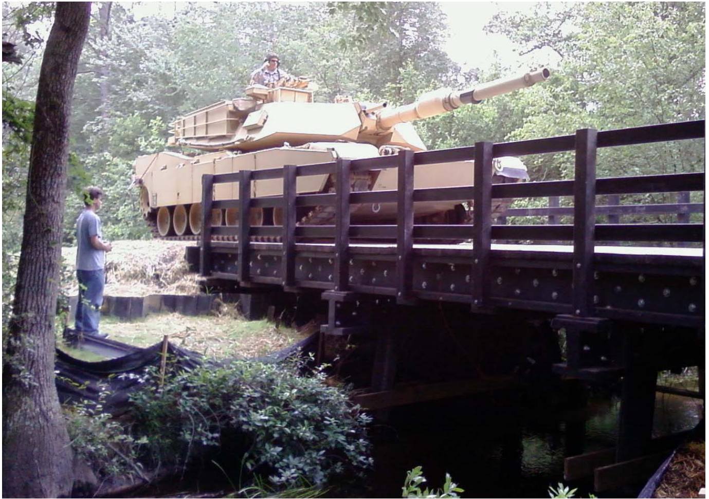
M-1 tank crossing the thermoplastic composite bridge during initial load testing
