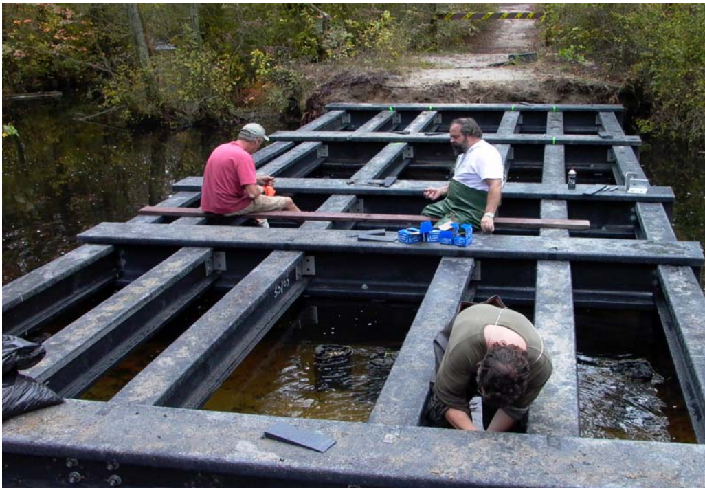
I-beam designed bridge being constructed at Wharton State Forest, NJ
