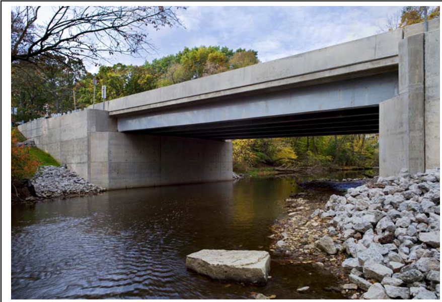
Fig 1 - 2008 ACEC Grand Award Winner – High Road Bridge over Long Run Creek First permanent HCB Highway Bridge funded by FHWA – IBRD Award
