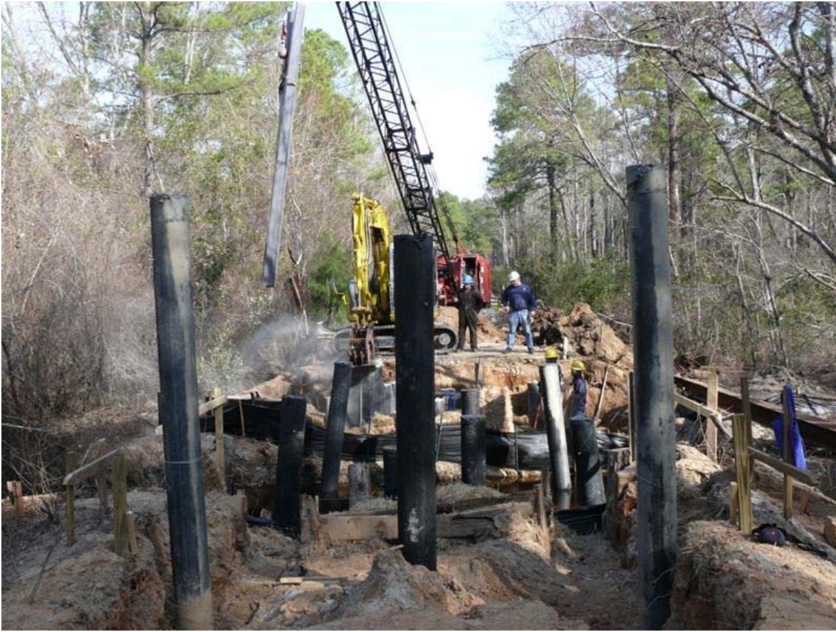
Thermoplastic Timber Pilings being driven at Ft. Bragg
