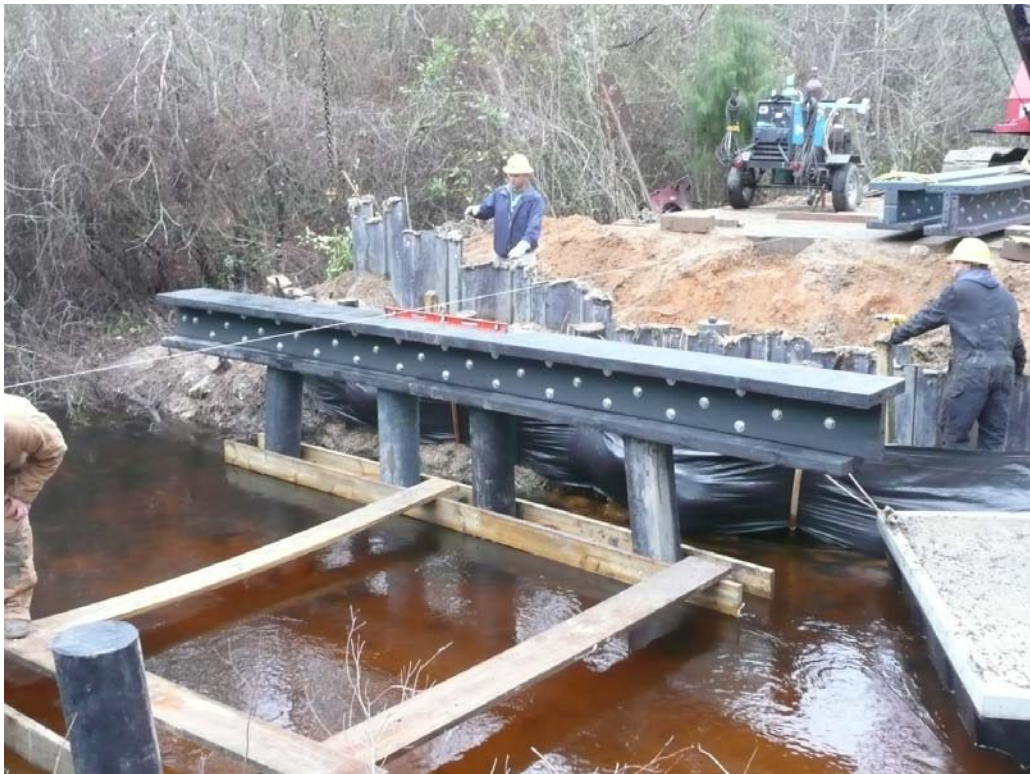
Construction of thermoplastic composite I-beam bridge at Fort Bragg.
