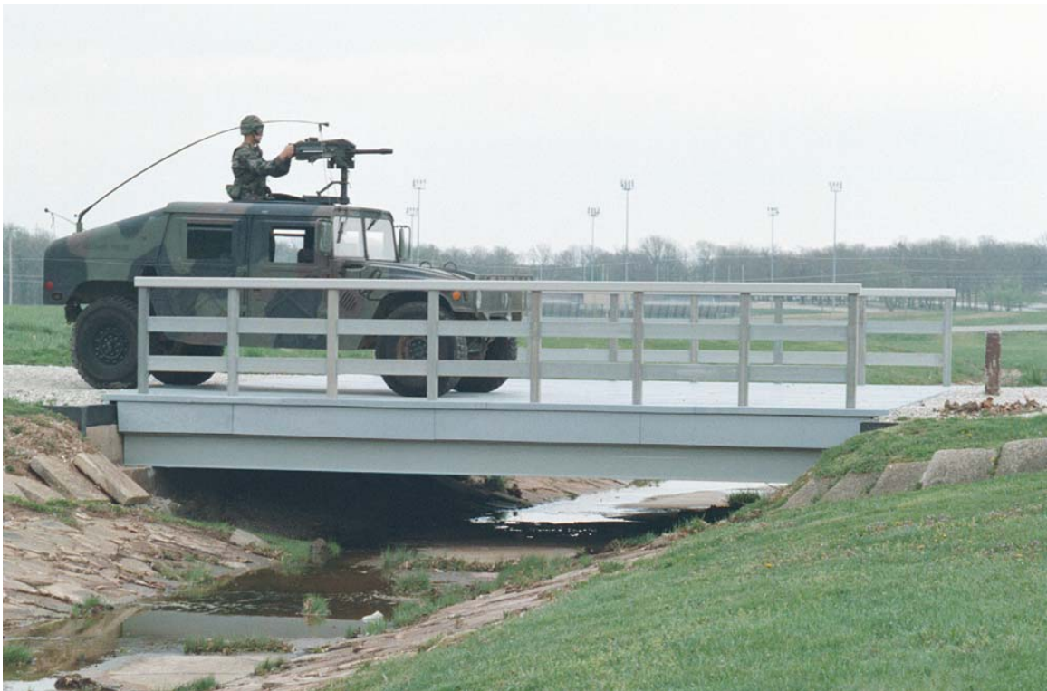
The first plastic lumber bridge built in the summer of 1998.
