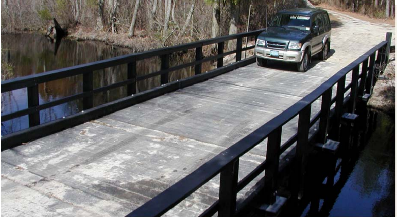
Finished I Beam Bridge at Wharton State Park. First Cost effective thermoplastic bridge
