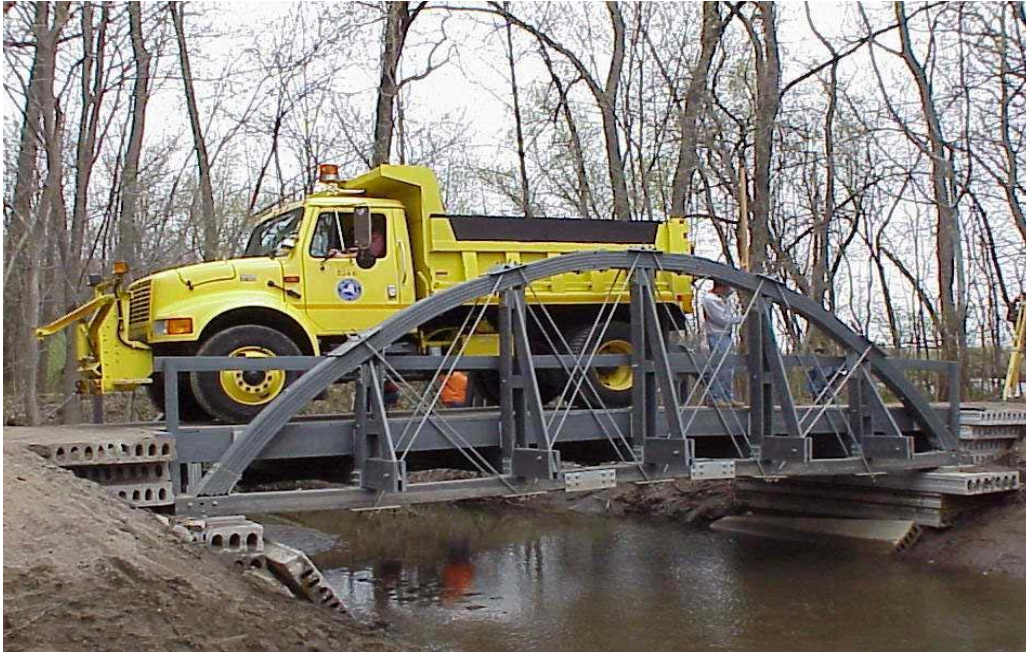
Load testing the plastic lumber, arch-truss bridge in Albany, NY.
