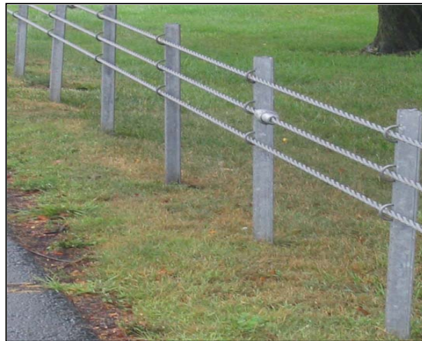
Figure 1. U.S. High Tension Cable System
