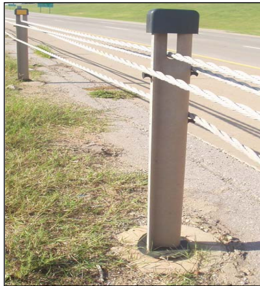
Figure 2. Brifen Wire Rope Safety Fence System
