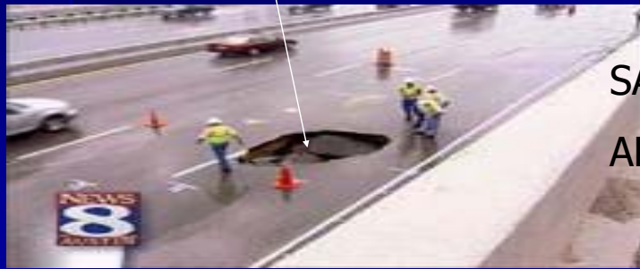
WATER MAIN BREAK UNDER INTERSTATE
