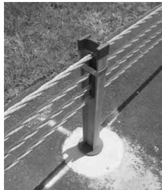
Concrete With Sockets
