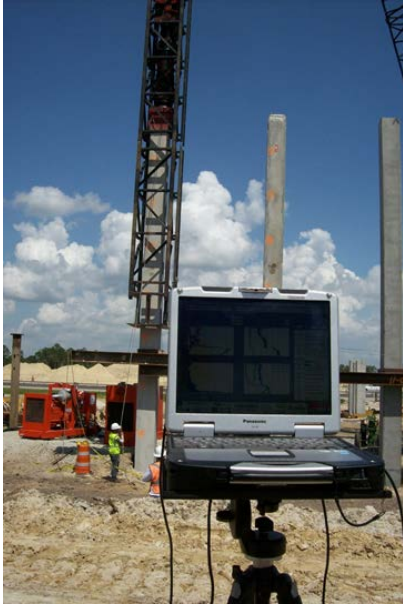
Embedded Data Collectors
