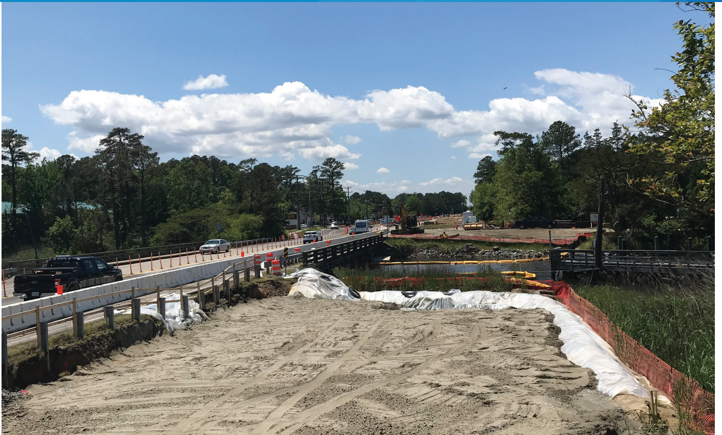
▶ This photograph shows construction work starting on the Laskin Road Bridge Replacement & Widening Project as this project was awarded in Fall 2019.
