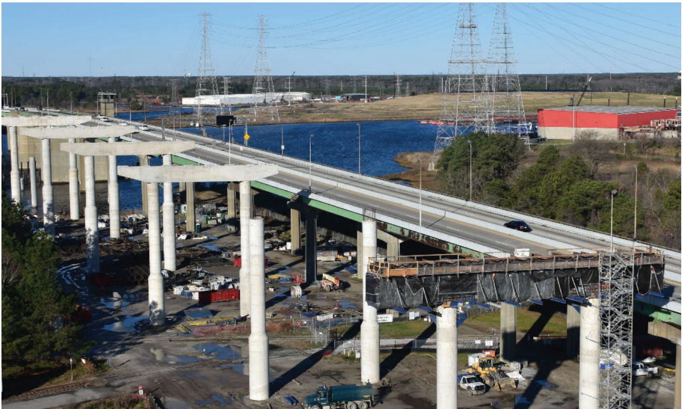
▶ This photograph shows construction underway on High Rise Bridge.
