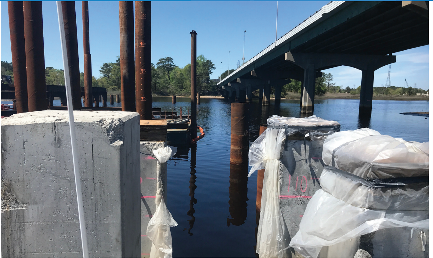
▶ This photograph shows precast concrete CFRP reinforced piles after driving. These piles are part of the High Rise Bridge with the CFRP used as the reinforcement for the 36-inch square prestressed concrete piles that are located in the water.
