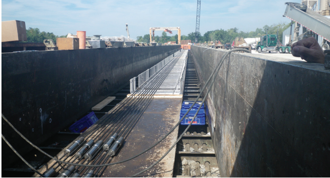
▶ Prestressed concrete box beam casting bed with hardened steel couples shown at photo bottom.
