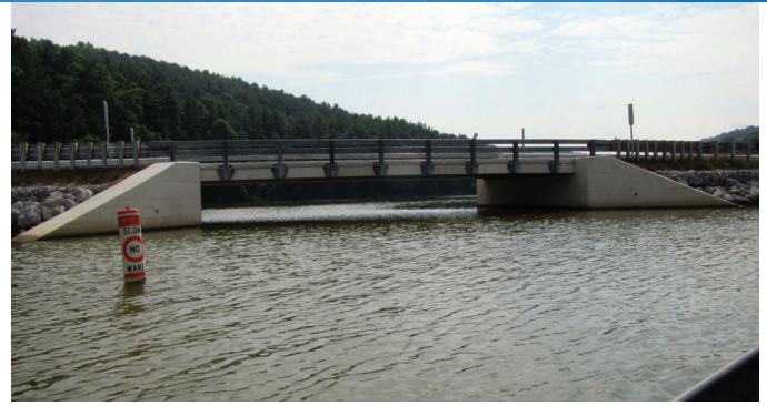
▶ Side view of completed bridge.
