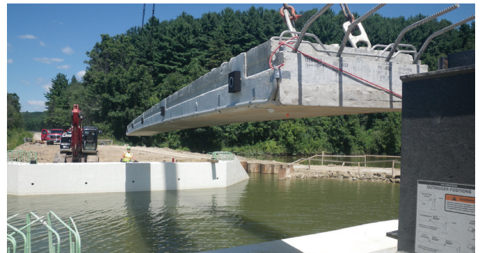
▶ Prestressed concrete box beam being launched onto the designated beam seat, the rectangular elastomers are for sealing the space between beams to allow for continuous grouting of the post tensioning duct.
