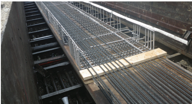
▶ Prestressed concrete box beam casting bed with the CFCC strand and the bottom stainless steel U-rebars used for shear reinforcement installed in place.
