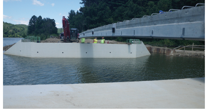
▶ An interior beam launching operation from the transporter to beam seat.
