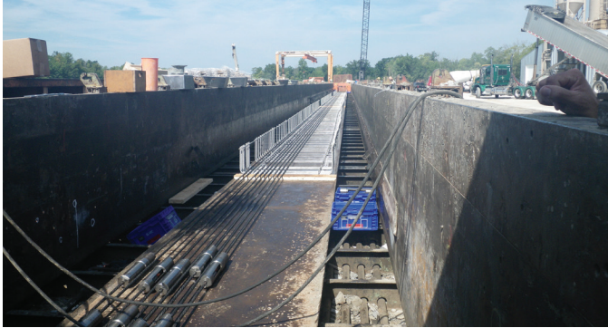
▶ Prestressed concrete box beam casting bed with hardened steel couplers shown at photo bottom.
