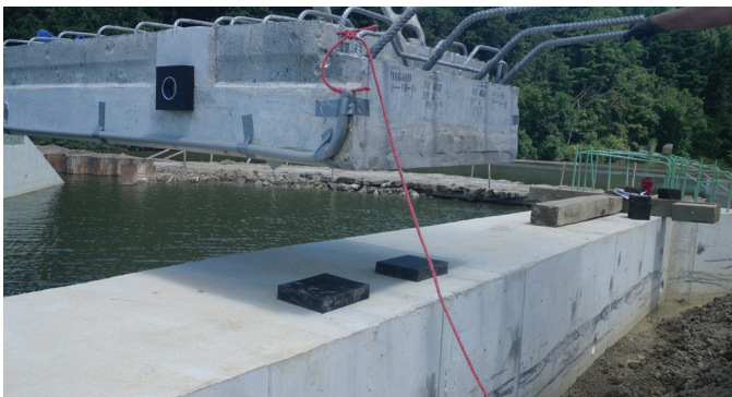
▶ Prestressed concrete box beam being launched onto the designated beam seat, the rectangular elastomers are for sealing the space between beams to allow for continuous grouting of the post tensioning ducts. The tubular foam at beam bottom is for sealing the edges to hold the grout between the beams.
