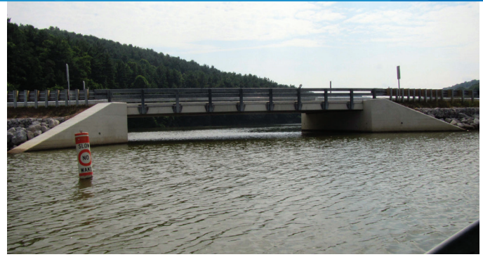
▶ Side view of completed bridge.
