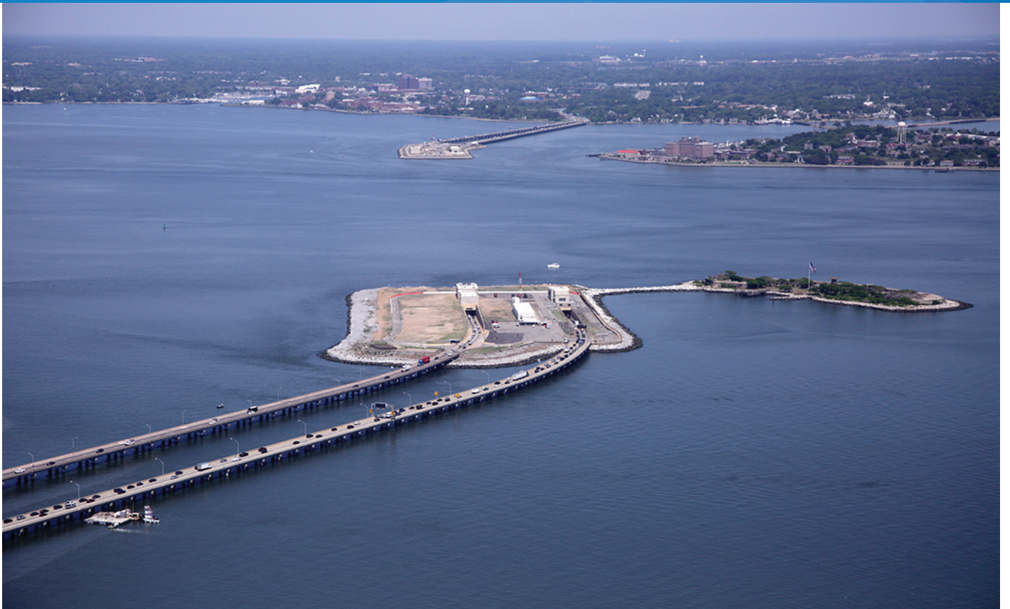
▶ This photograph shows the structures leading to the tunnels and open shipping channel.
