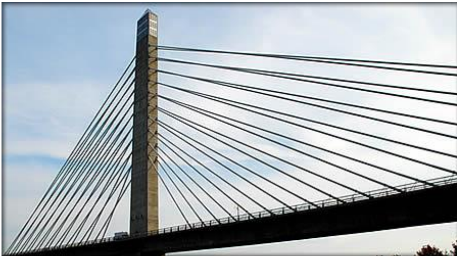
Maine Cable Stayed
