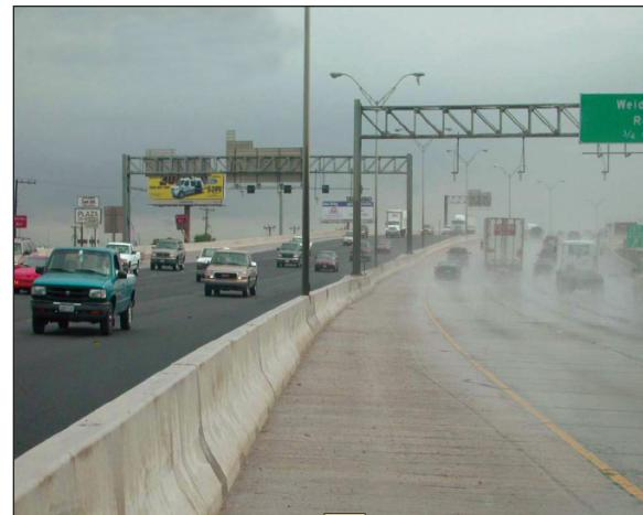
*The use of permeable friction course (installed on the roadside to the left) reduces splash and spray.*
