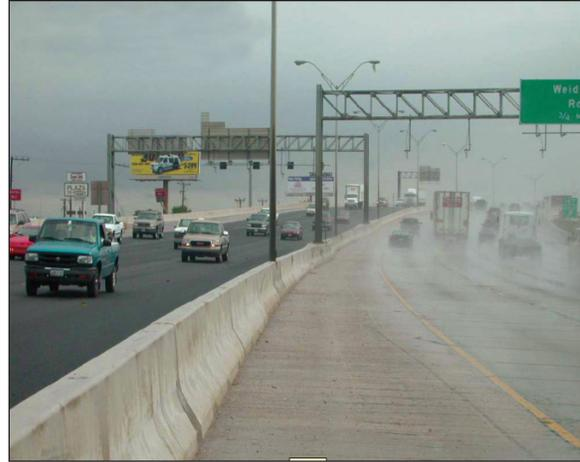
*The use of permeable friction course (installed on the roadside to the left) reduces splash and spray.*
