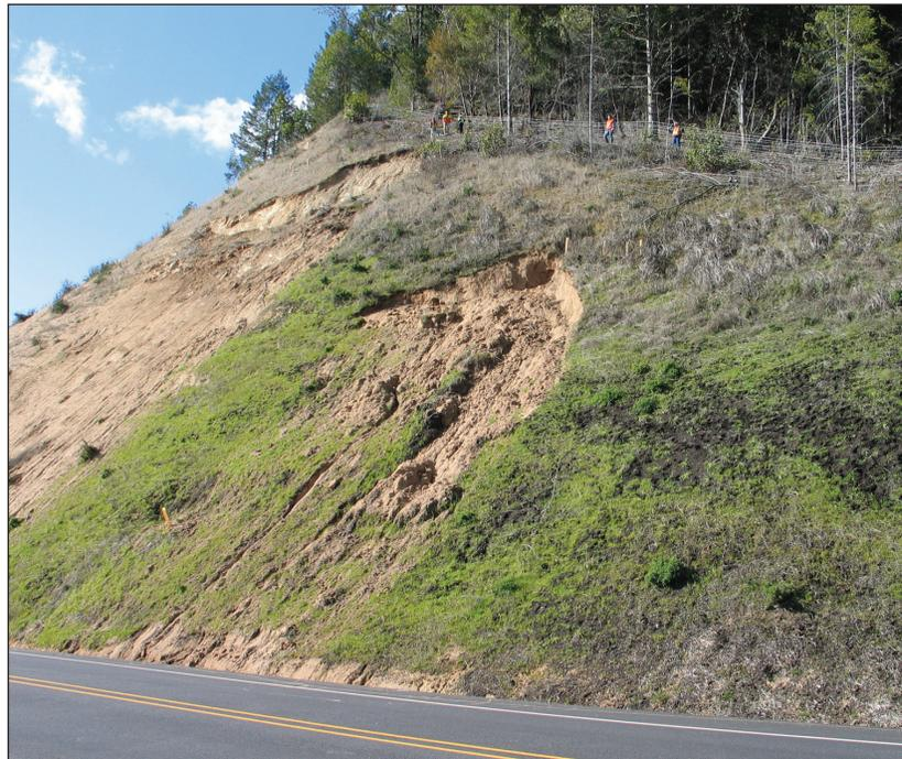
*This debris slide took place two years after construction, when grasses were fully established. To preclude these kinds of problems, revegetation should have the establishment of long-term plant communities, not just quick cover, as a goal.*
