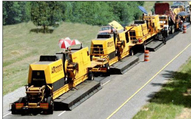
Hot In-Place Recycling Paving Train Including Multiple Pavement Heaters. Photo: American Recycling and Reclamation Association.
