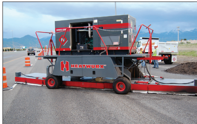
Hot In-Place Recycling Pavement Repair Equipment.
