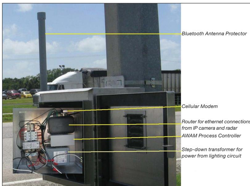
An AWAM sensor field installation. The equipment installed on IH45 to Dallas was deployed to monitor traffic during a hurricane evacuation event.
