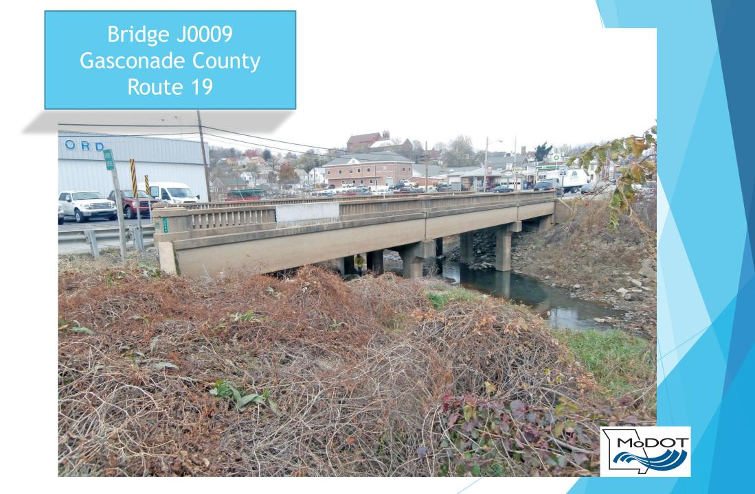
U.I.P. AND MODIFY EXISTING SUBSTRUCTURE AND REPLACE SUPERSTRUCTURE WITH (32')(42.5')(42') SIMPLE COMPOSITE 18" PRESS BRAKE FORMED TUB GIRDER SPANS
