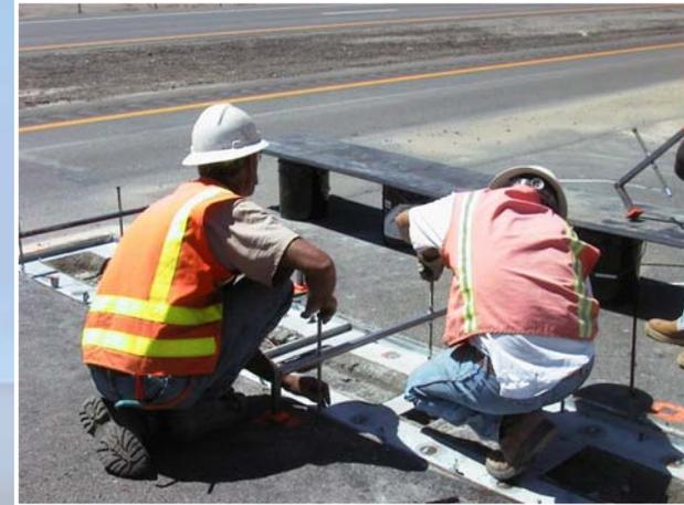
Nevada DOT installs WIM bending plate in PCC Portland Cement on I-80 near Verdi, NV
