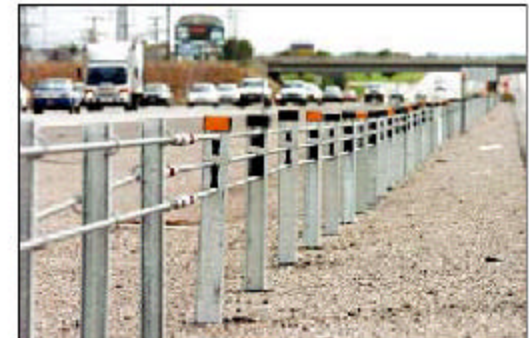
Freeway cable barrier on I-215 near the E-Center is made of three high-tension cables that may save lives.
