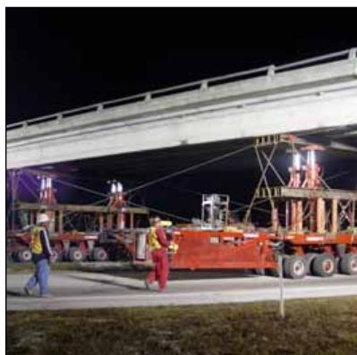
Workers walk along a SPMT used to move a section of the Graves Avenue Bridge during a project in Florida in 2006.
