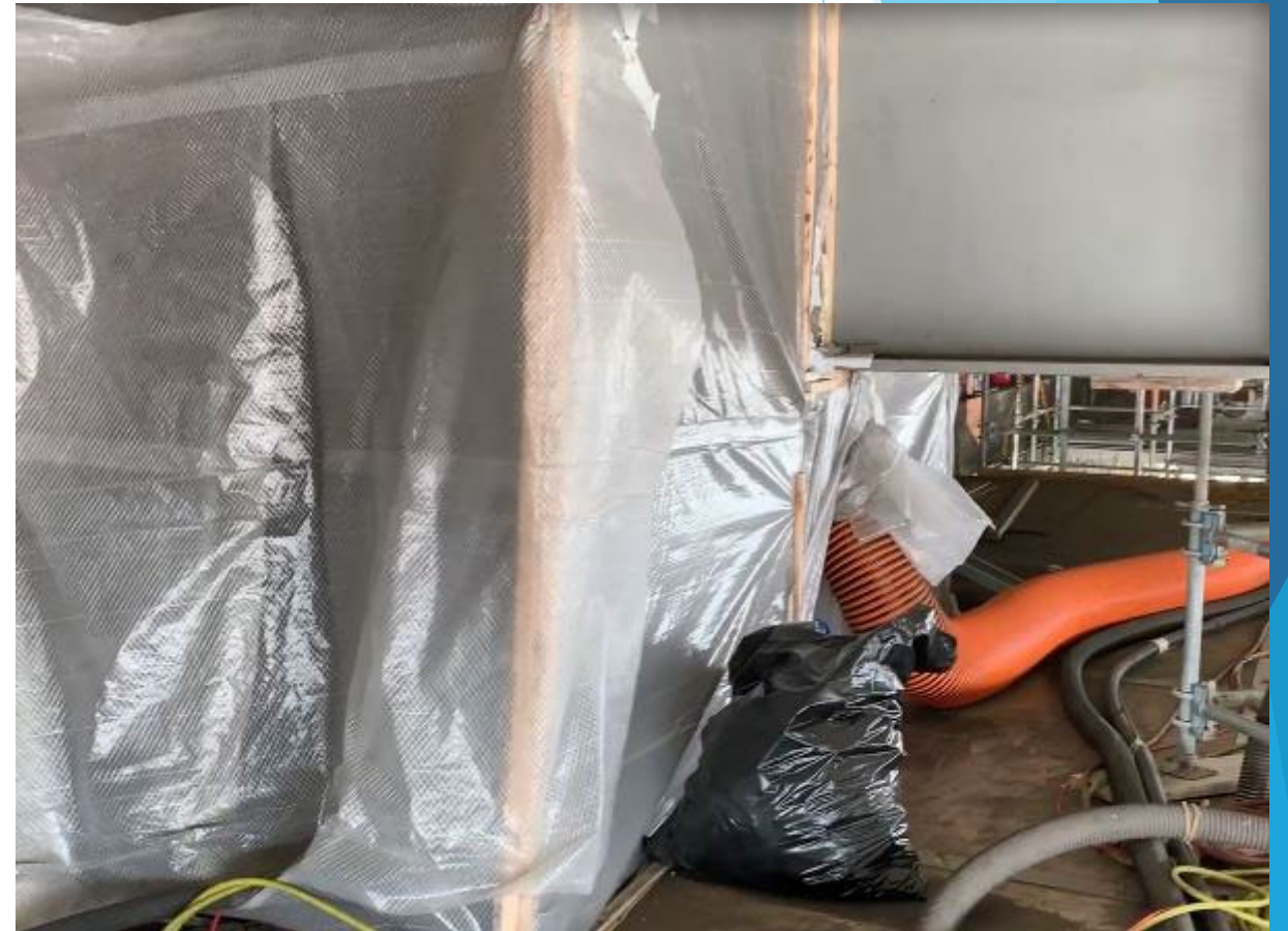
Sandblasting with Lead Abatement
