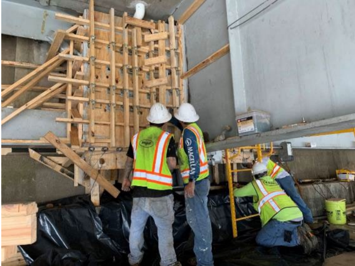
Under the Deck
