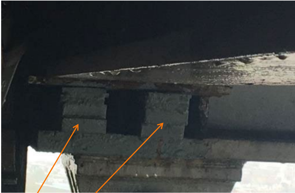
Shim Plates Installed (All Bearings)
