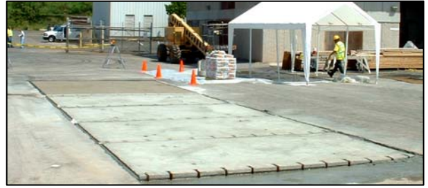
KWIK SLAB system installed in existing asphalt paving.
