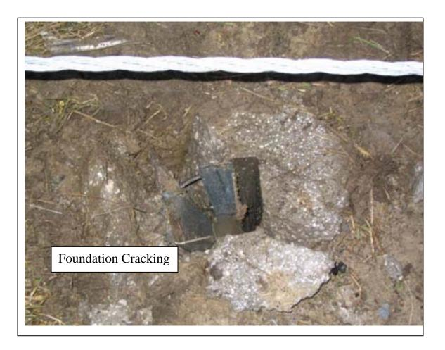
After some of the terminal end foundations were put under a load, it was noted that end anchors appeared to be rotating out of the ground. It was suspected that this problem was also due to soil conditions. Brifen indicated that these types of failures have not been a problem on other WRSF installations. However, a report from Iowa reported that they had experienced this problem but it was not widespread.
