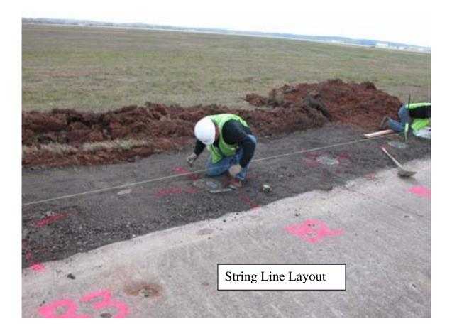
Line post holes and end terminal foundations were 30 inches deep. Using the string line for reference, the foundation holes were cored to the proper depth every 10.5 feet along the run. The line post foundations were 12 inches in diameter and the end anchors were 48 inches in diameter. A one ton truck with an auger was used for excavating. Waste soil was distributed along the median manually or removed using a Bobcat (small earth mover).
