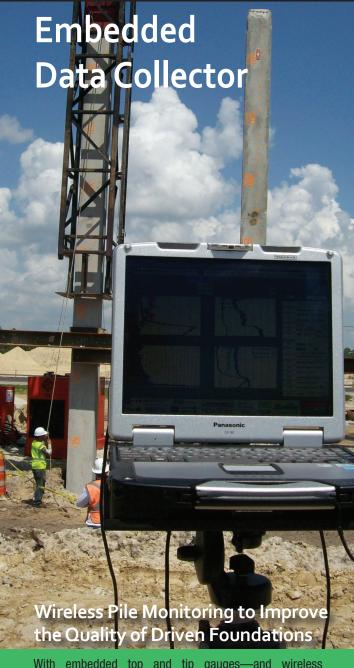
With embedded top and tip gauges—and wireless communication in real time to a laptop onsite—operators can achieve a more accurate assessment of side friction and tip components when driving prestressed concrete piles.
