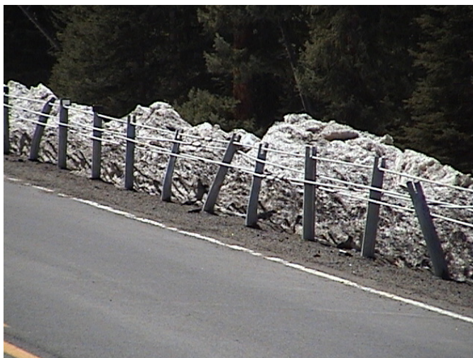
Figure 5. Posts on SH-65 are bent in all directions, suggesting that the damage is not all caused by snowplows.
