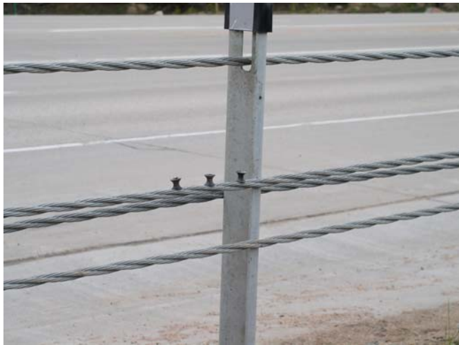
Figure 6. Cables positioned lower than design height.
