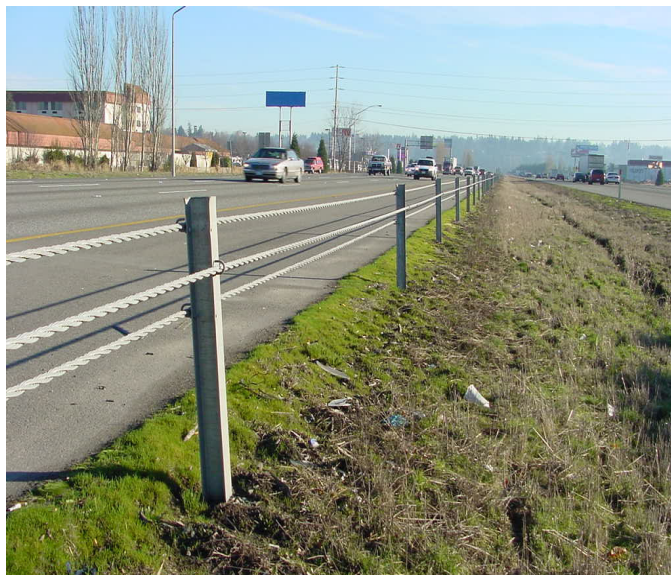
FIGURE 1 Typical cable median barrier installation and details
