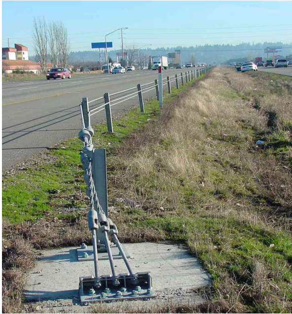
FIGURE 2 Washington State cable barrier terminal
