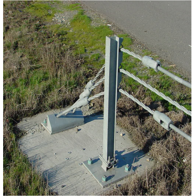
FIGURE 2 Washington State cable barrier terminal
