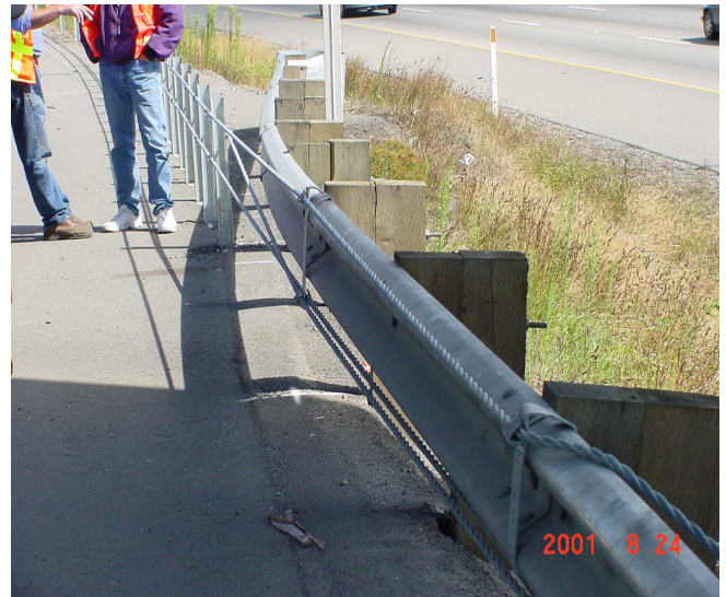
FIGURE 2 Washington State cable barrier terminal
