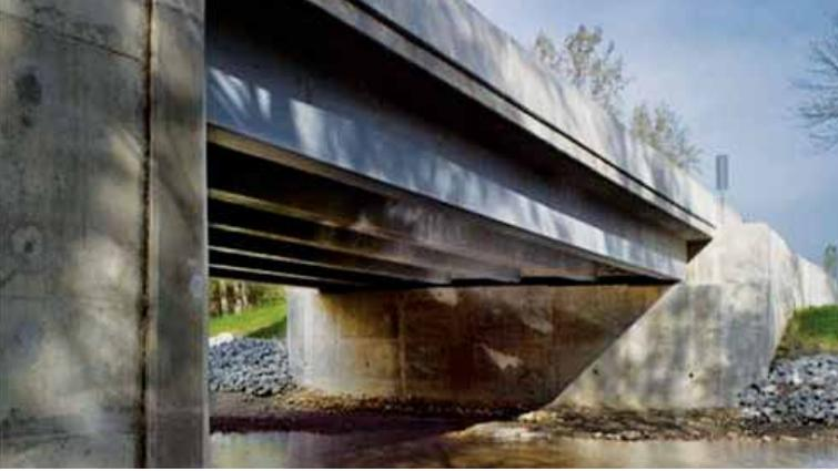
**Hybrid-Composite Beams (HCB)** have the potential to be long-lasting, can weigh considerably less than standard concrete beams, and may be placed using smaller, lighter pieces of construction equipment. They show promise for long service life with corrosion resistance, and can provide a low overall
