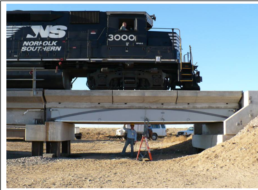
Fig 4. Nov 2007 – TTCI, Pueblo, CO. World's first Composite Railroad Bridge, constructed with HCB's developed with funding from TRB, High Speed Rail-IDEA Program. Endurance testing to date includes over 95 million gross tons (MGT) of heavy axle railroad loading.
