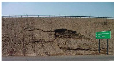
Surficial slope failures (nuisance slides) constitute a significant economic and manpower burden for many transportation agencies due to the frequent and recurring nature of the slides. A new, cost-effective alternative for stabilizing these slopes was desired.
