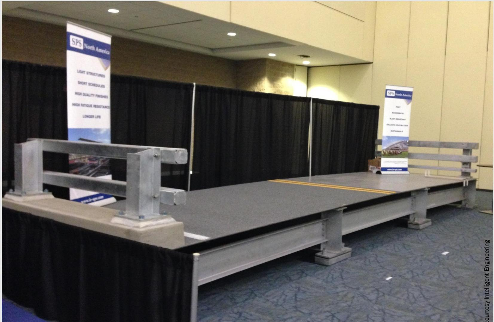
Modular bridge section illustrating TL2 and TL4 guardrail systems
