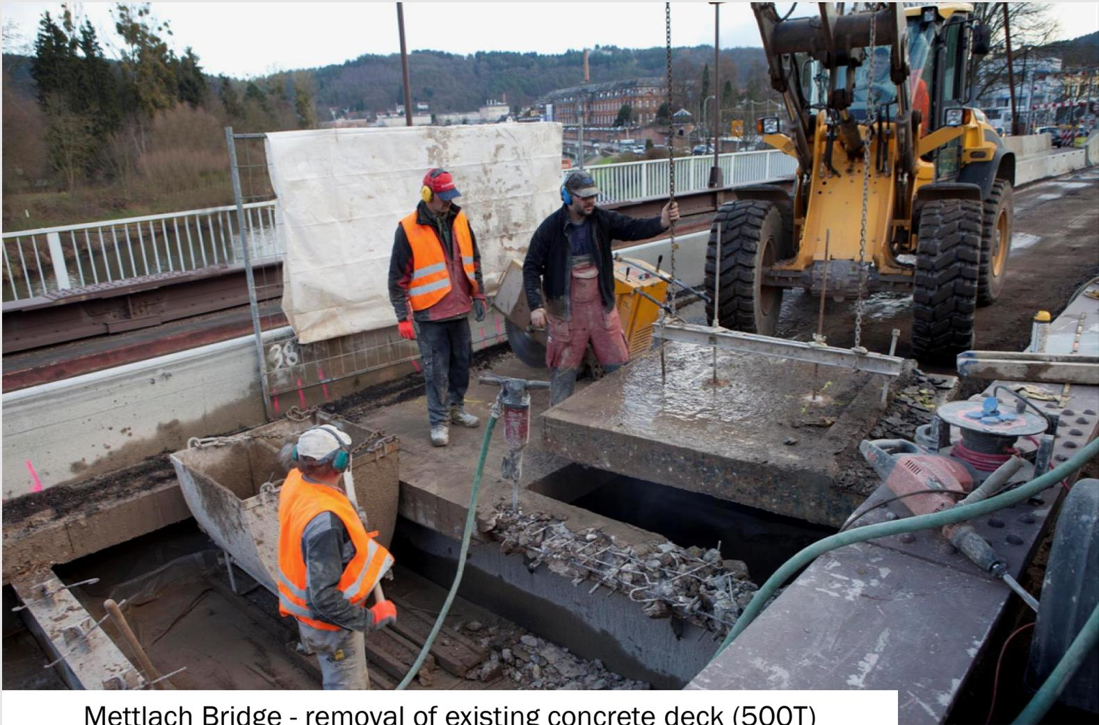
Mettlach Bridge - removal of existing concrete deck (500T)
