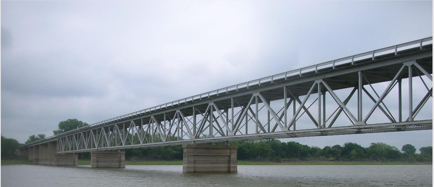
SPS reduces the deck dead load by over 50% from 100 lbs/ft (8" concrete deck) to 45 lbs/ft (SPS)
