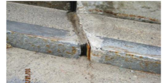
The joint seal splices (left photo) seem to be holding up well. The seal is supplied in 6.56 LF (2 m) lengths and is bonded end to end in the field with a silicone adhesive prior to insertion into the joint. The silicone sealant bead that runs the length of the seal and bonds to the steel is still holding up well for the most part.
